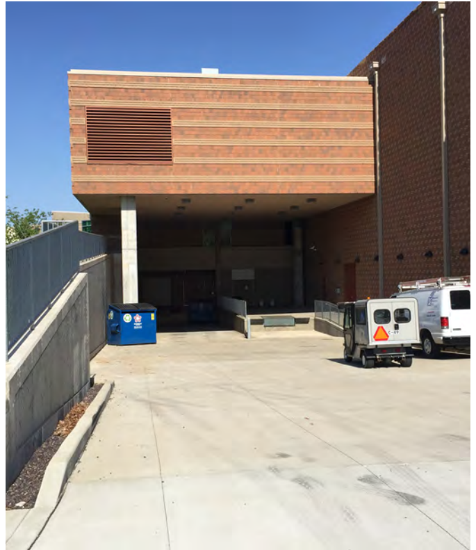
Existing Loading Dock
