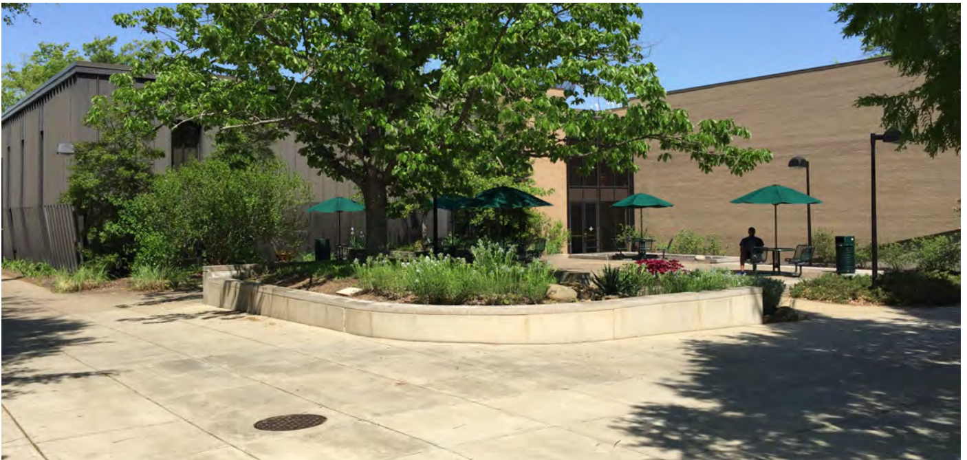
Existing Entry Courtyard
