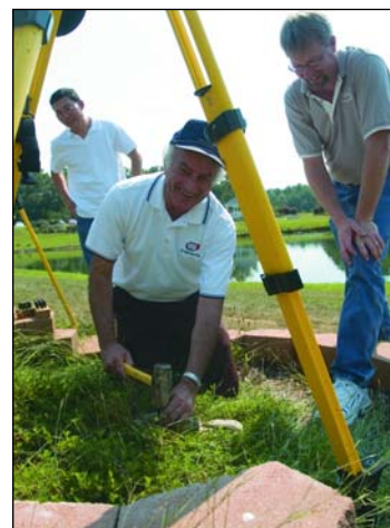
Jack Naghdi, kneeling, applies his initials to the new GPS control point on campus while former USI student Doug Bacon, right, of Morley and Associates and current surveying students look on.
